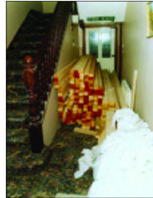
Figure 9: A blocked corridor with incorrect signage
