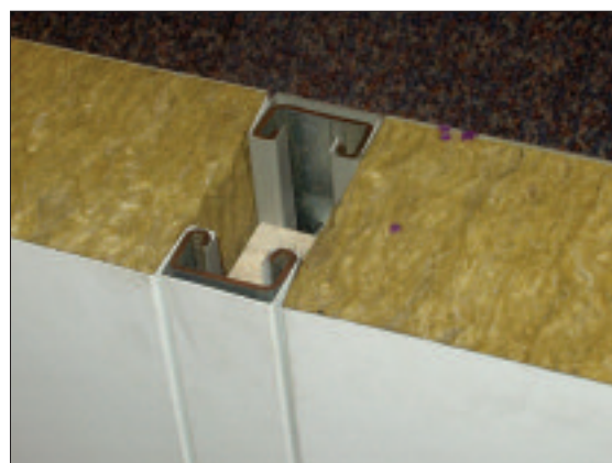
Figure 17: Insulated core panels – internal
